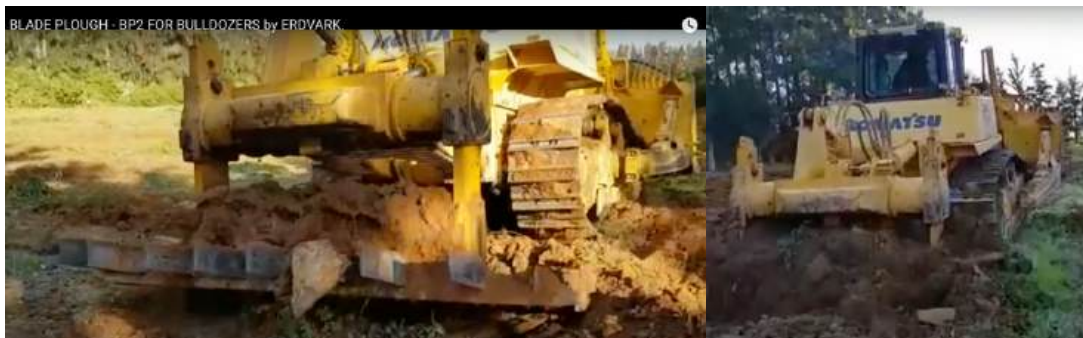
Fig 11 Erdvark BLADE PLOUGH behind dozer
