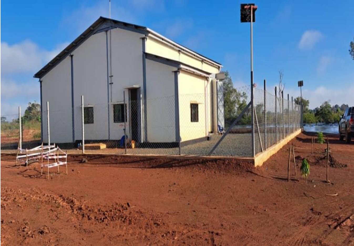
Final establishment of Irrigation room as part of intake -1
