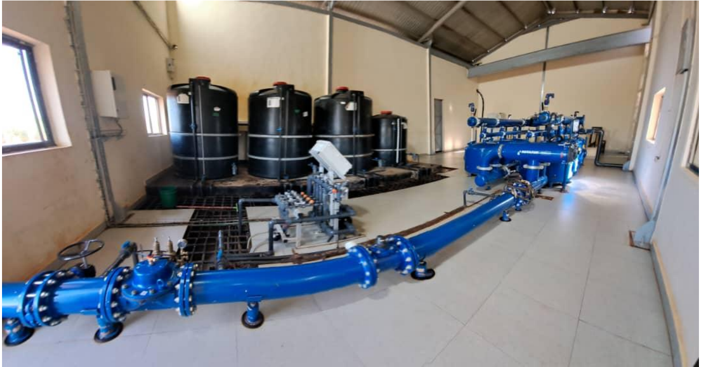
Inner view of Irrigation room in Intake-1
