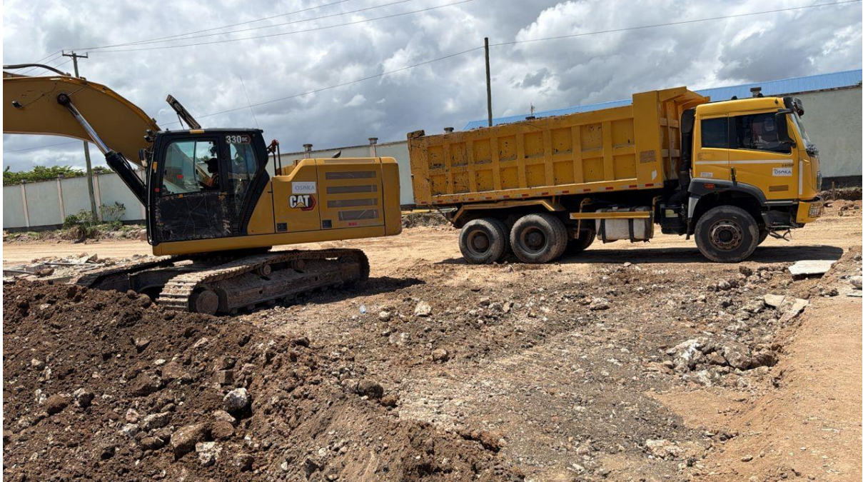
Figure 01: cutting to spoil area II
