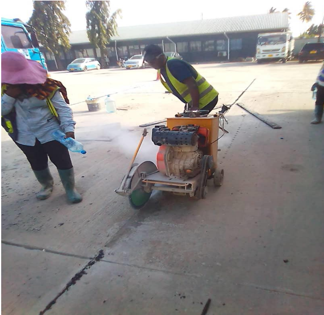
Figure 04: Joint cutting and sealing area III
