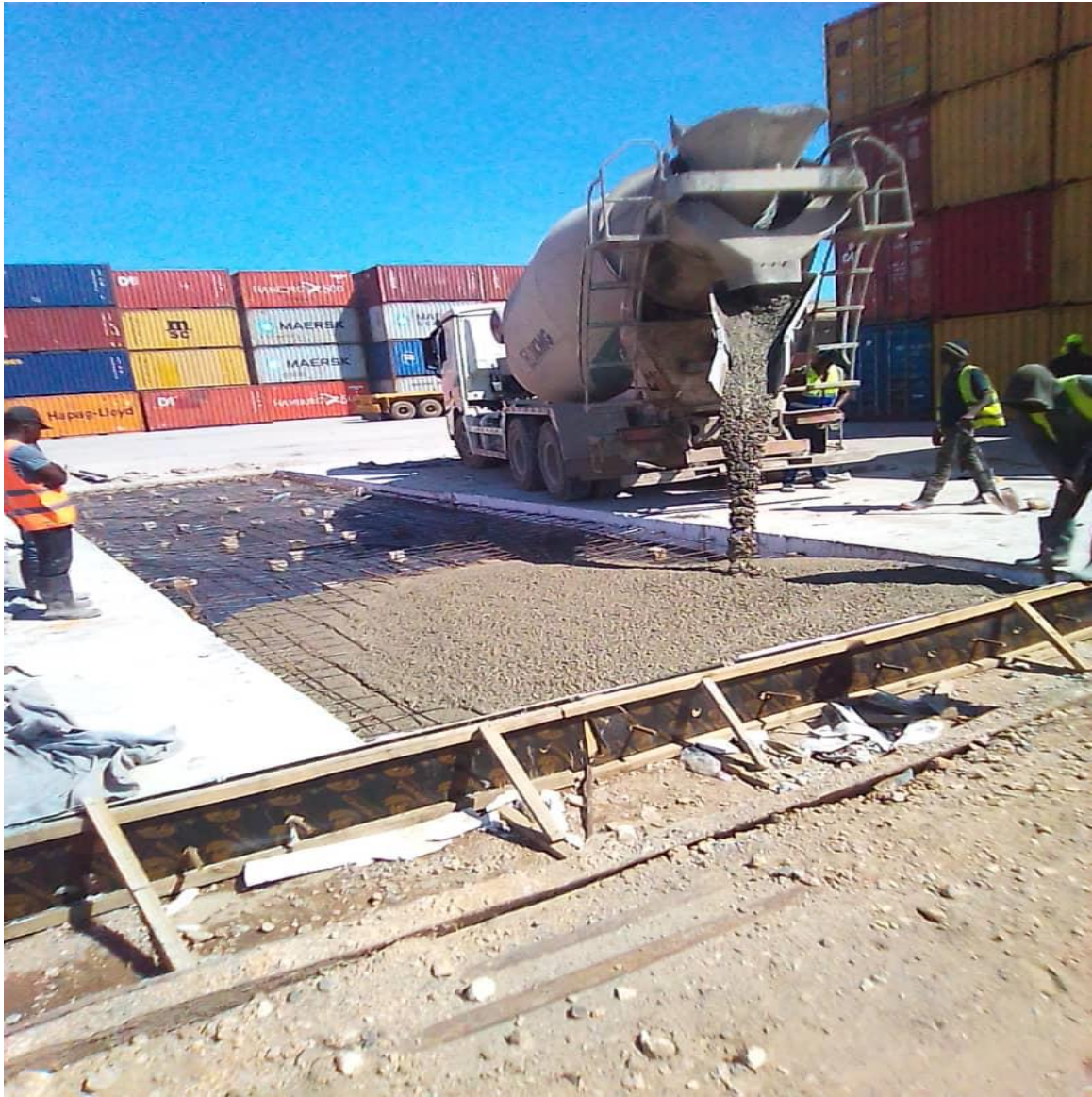
Figure 08: Concrete casting area I
