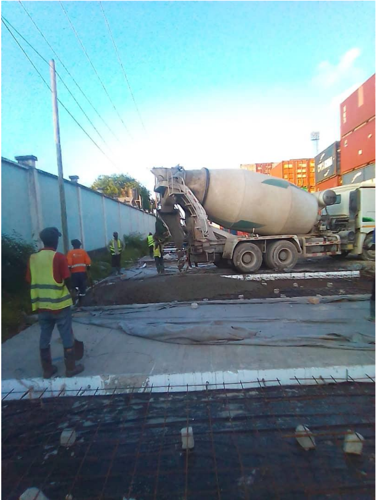
Figure 06: Concrete casting area IV C
