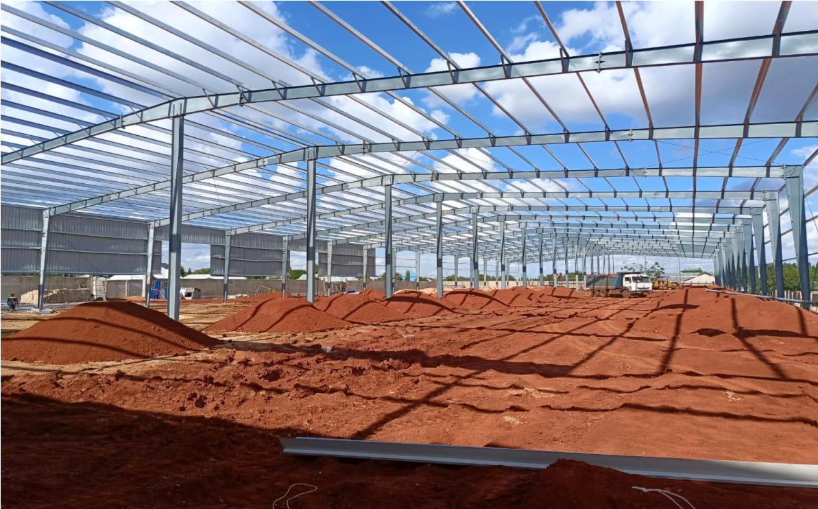
Undergoing levelling and Base formation during structure erection;
