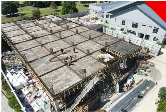
Image 1: Construction of the Factory at Ununio.
