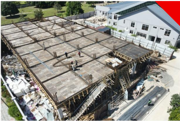
Image 1: Construction of the Factory at Ununio.
