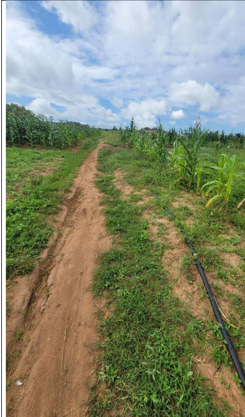
3-kms long Irrigation Pipe
