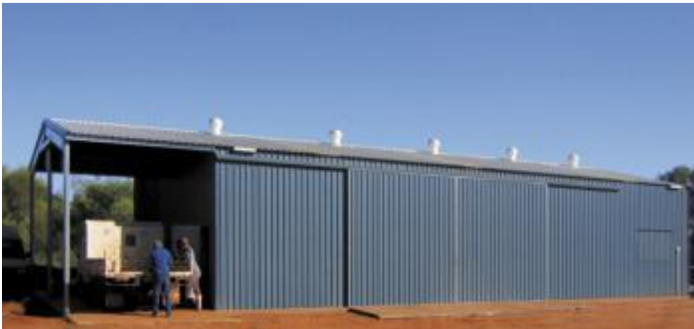
Example of Stage 1 warehouse inside of which the initial cold store would be placed to reduce energy usage.
