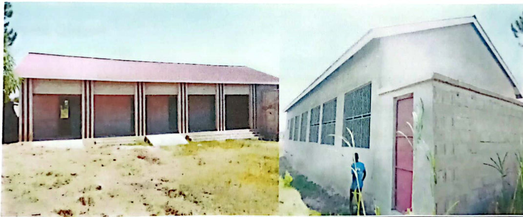
View of the Baking Building
