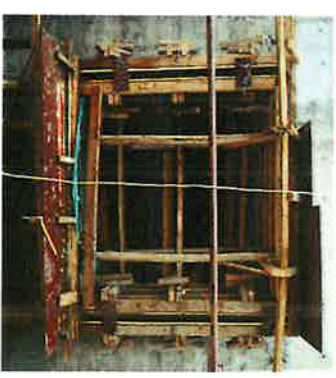
Mockup in progress
