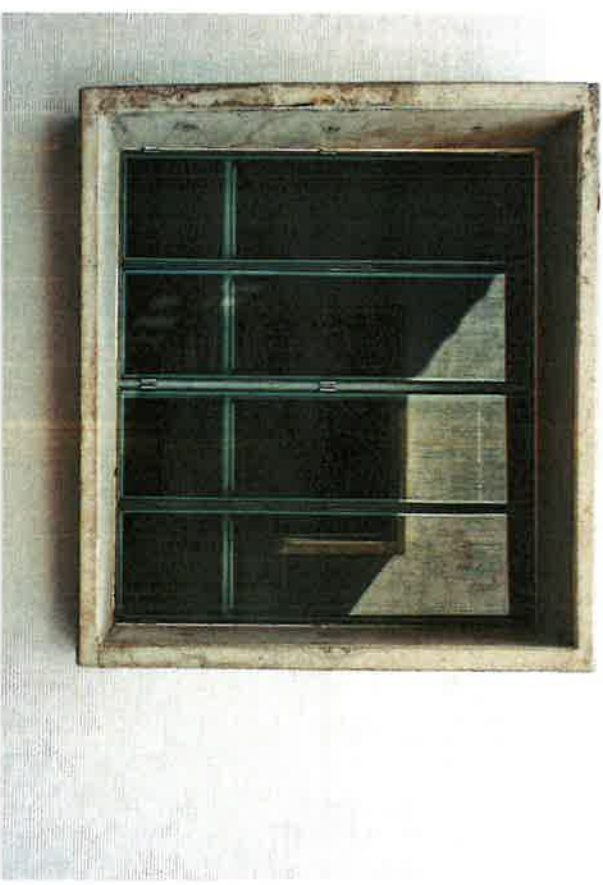
Window shading box textured wall plaster
