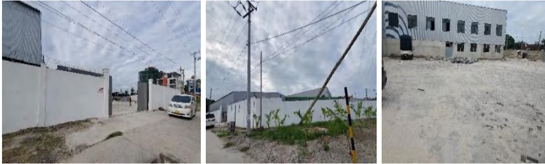
General overview of the plot and site works
