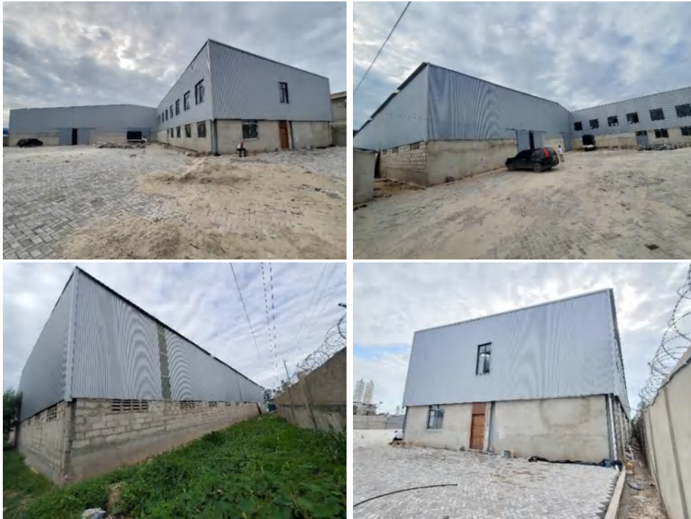
Different elevations of the Main Building
