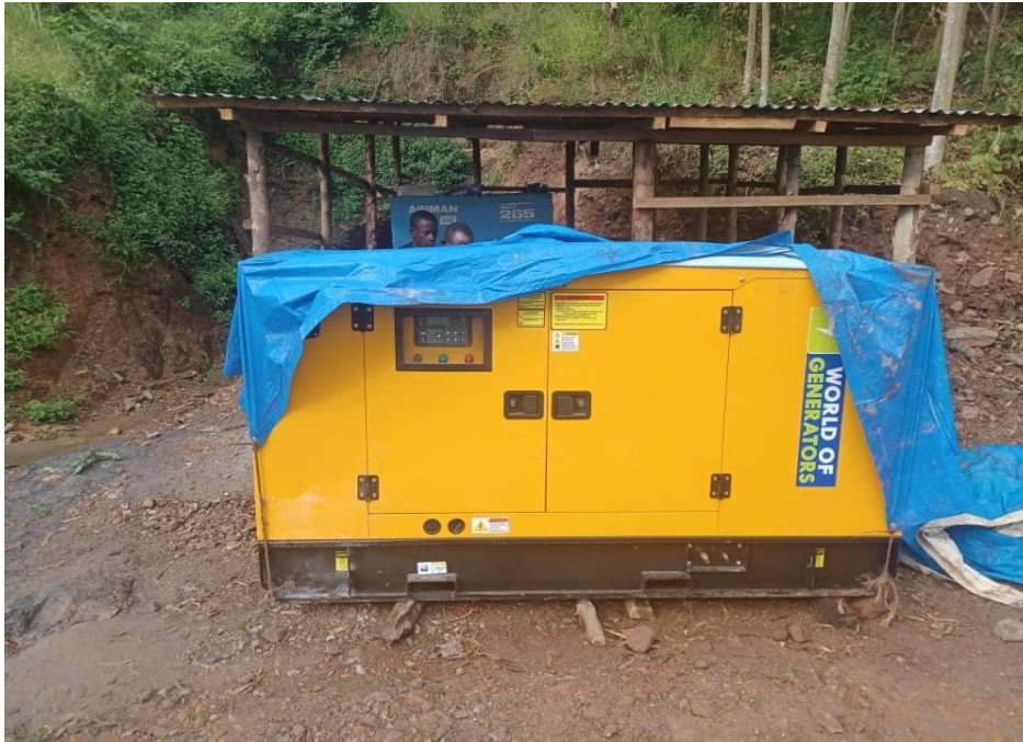
Figure 1. Generator KVA 60
