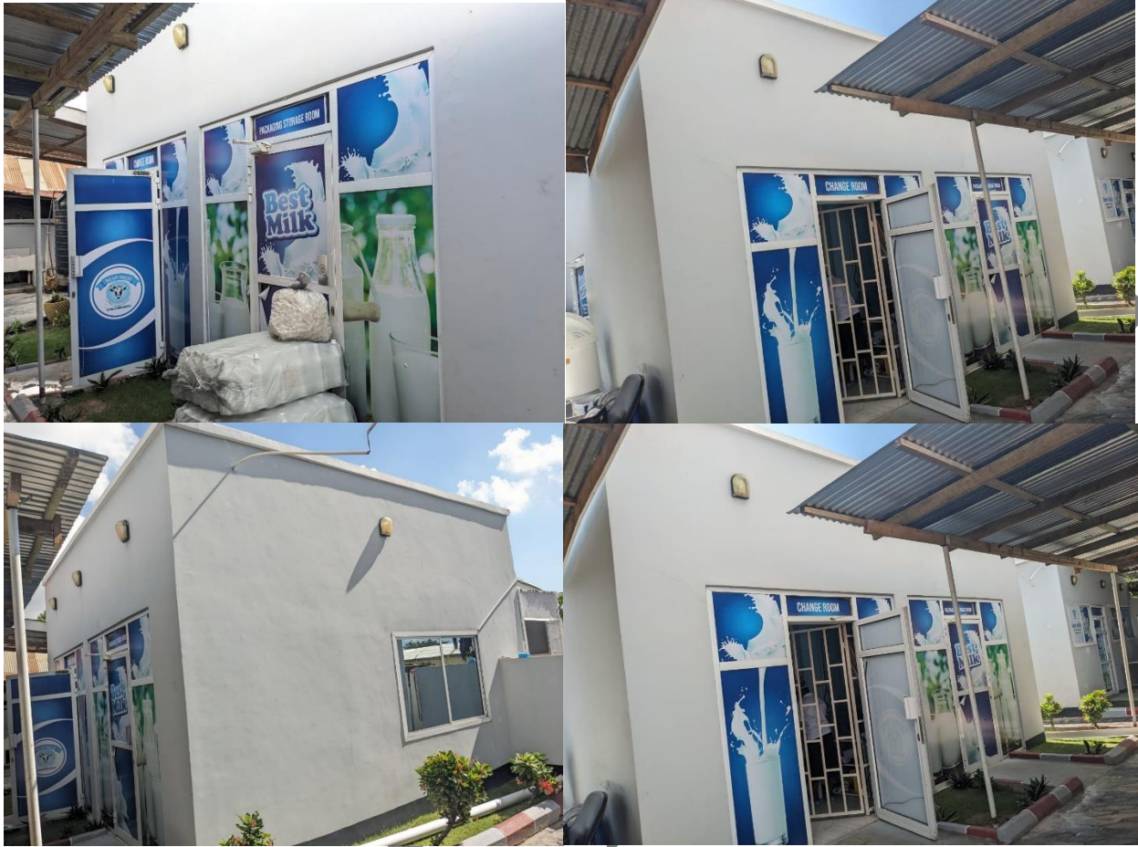
General View of Main building
