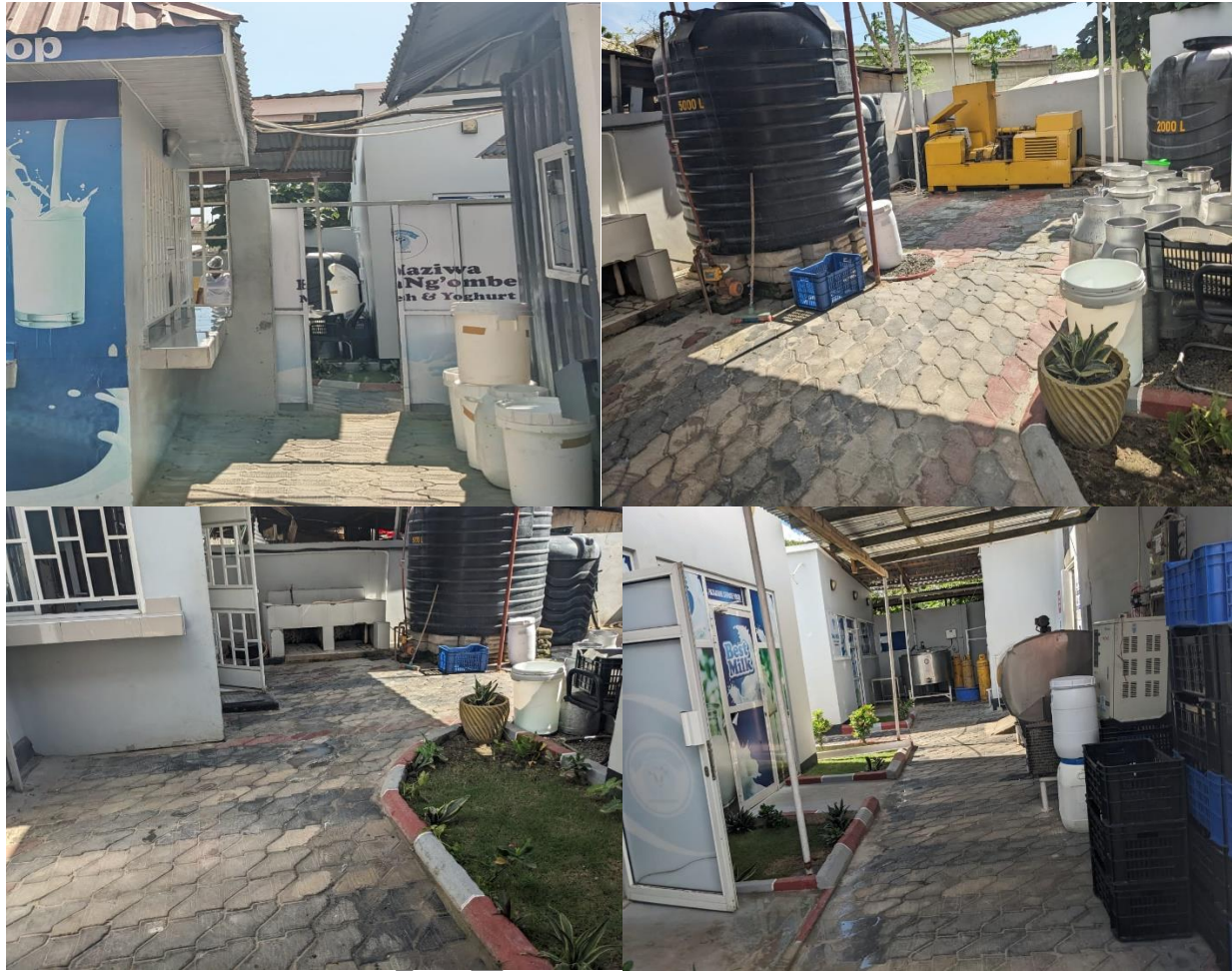
General view of Siteworks
