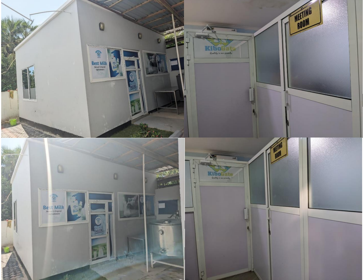
General View of Office Building
