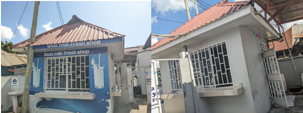
General View of Shop frame
