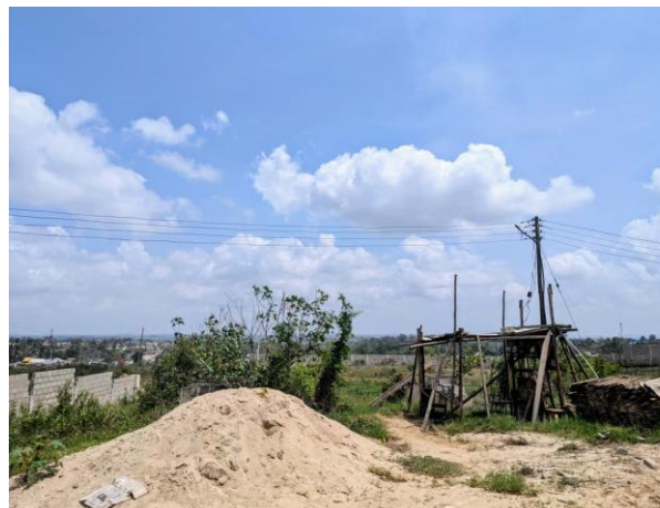
Constructed fence surrounding project area
