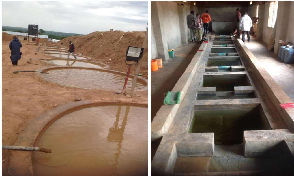
Fig. 1.3 - 2: Typical VAT Leaching Project in Geita for Mr. Ngala Saguda Ndulu
