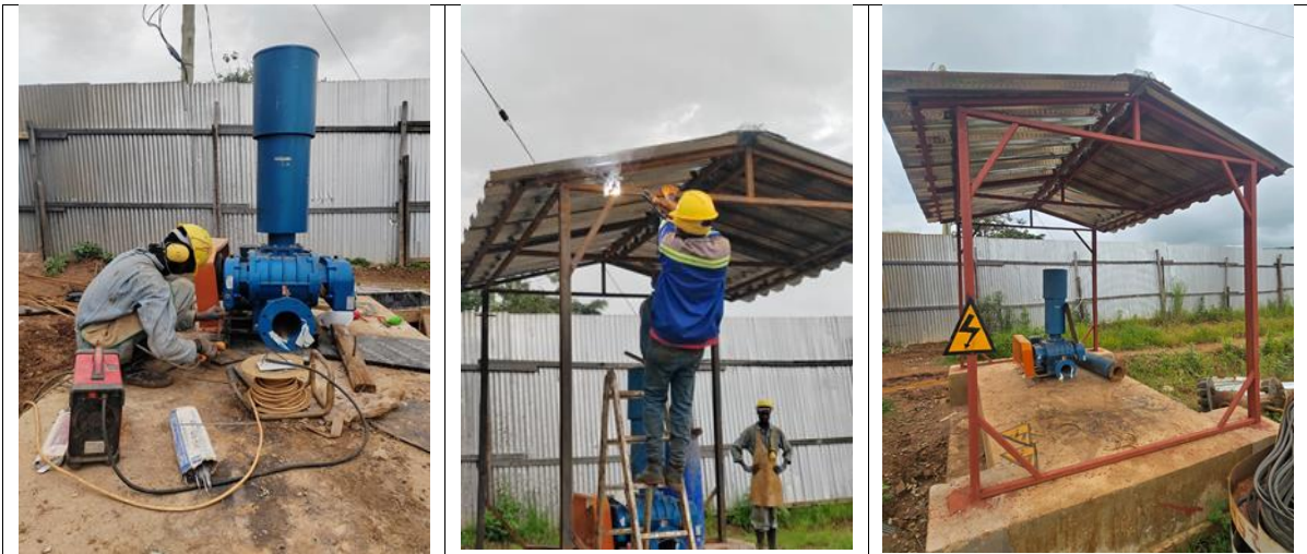
Construction and Installation of Root Blower
