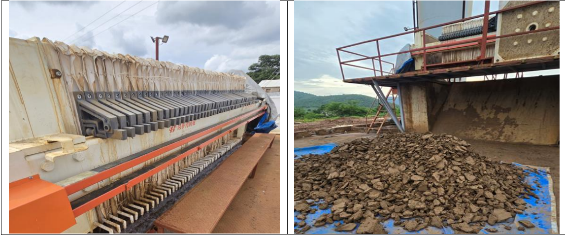
Filtration System Installation and Operation
