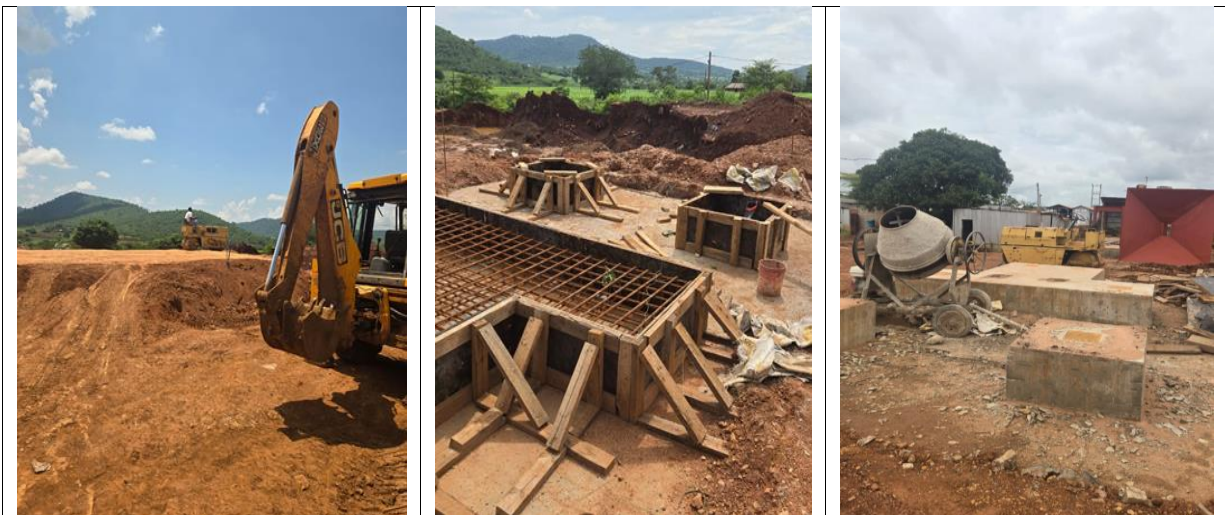
Crusher System Installation
