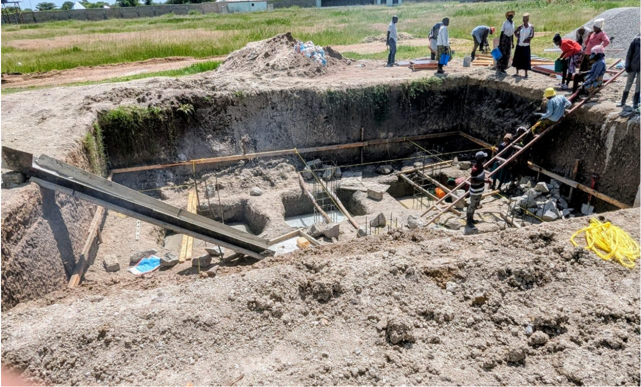
The area where a solvent plant machine will be installed.
