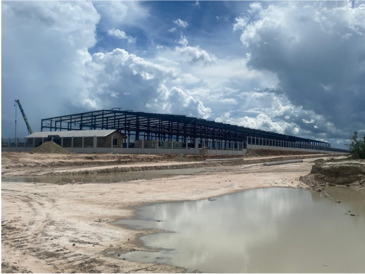
Figure 2: The building in construction at Kwala Industrial park
