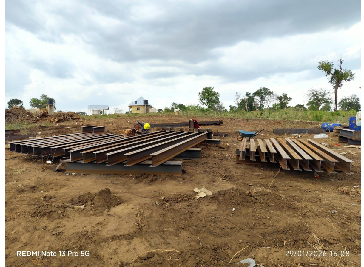
Hydro cyclone structure work in progress
