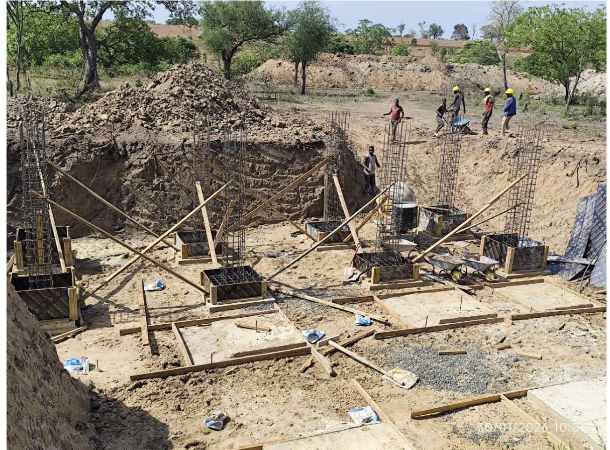
GC Unit steel alignment
