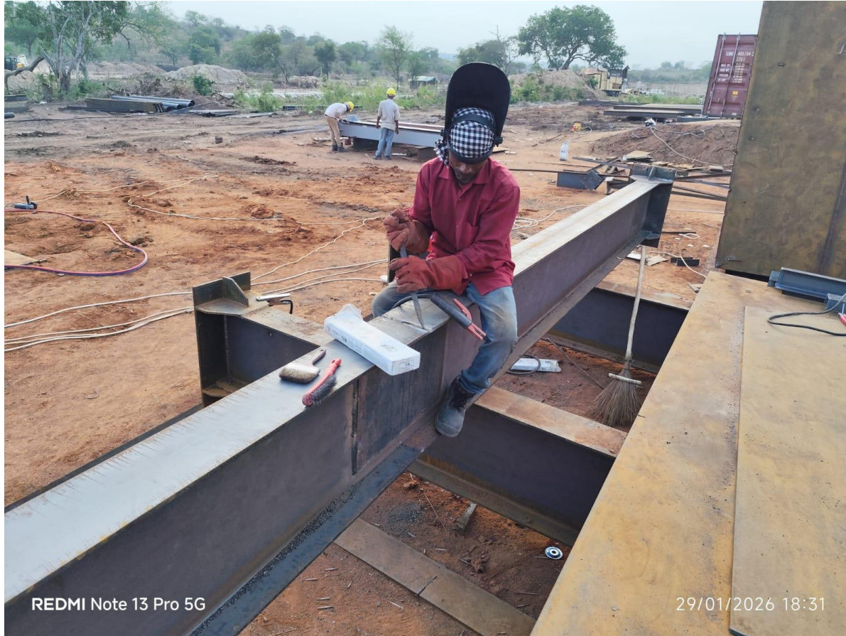
Columns full welding in progress
