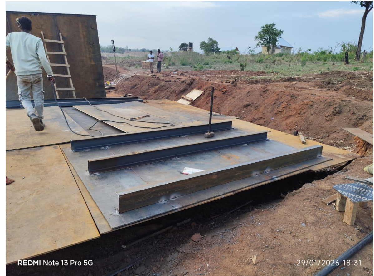
Hammer crusher slurry tank plates Notch cutting & Fitting
