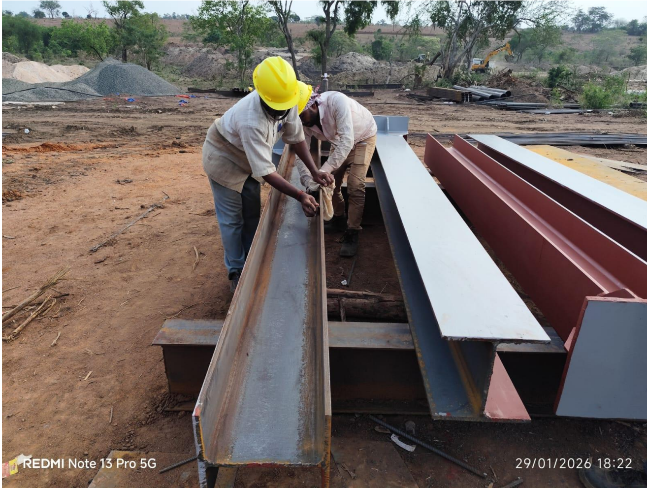
Structure paint preparation
