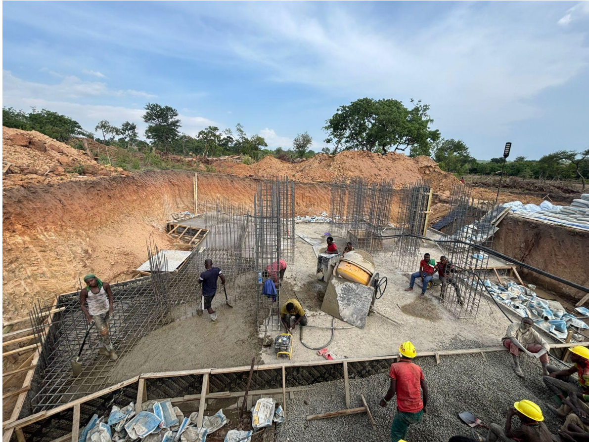
Crushing unit concreting work
