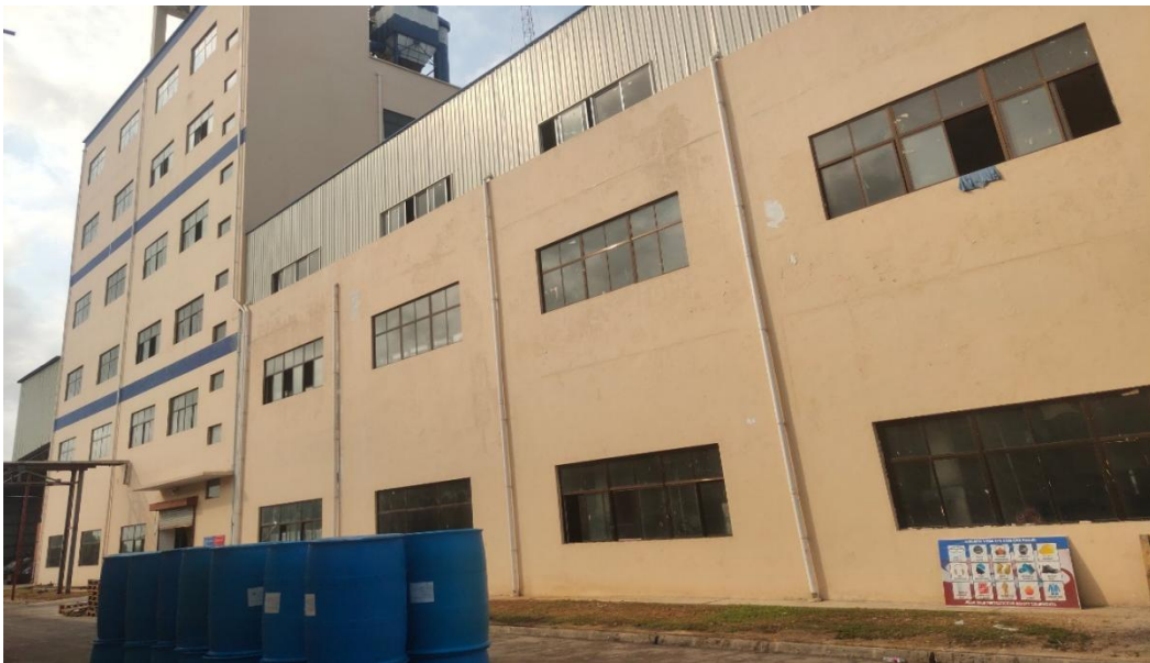
Picture No 1. Outside of the factory
