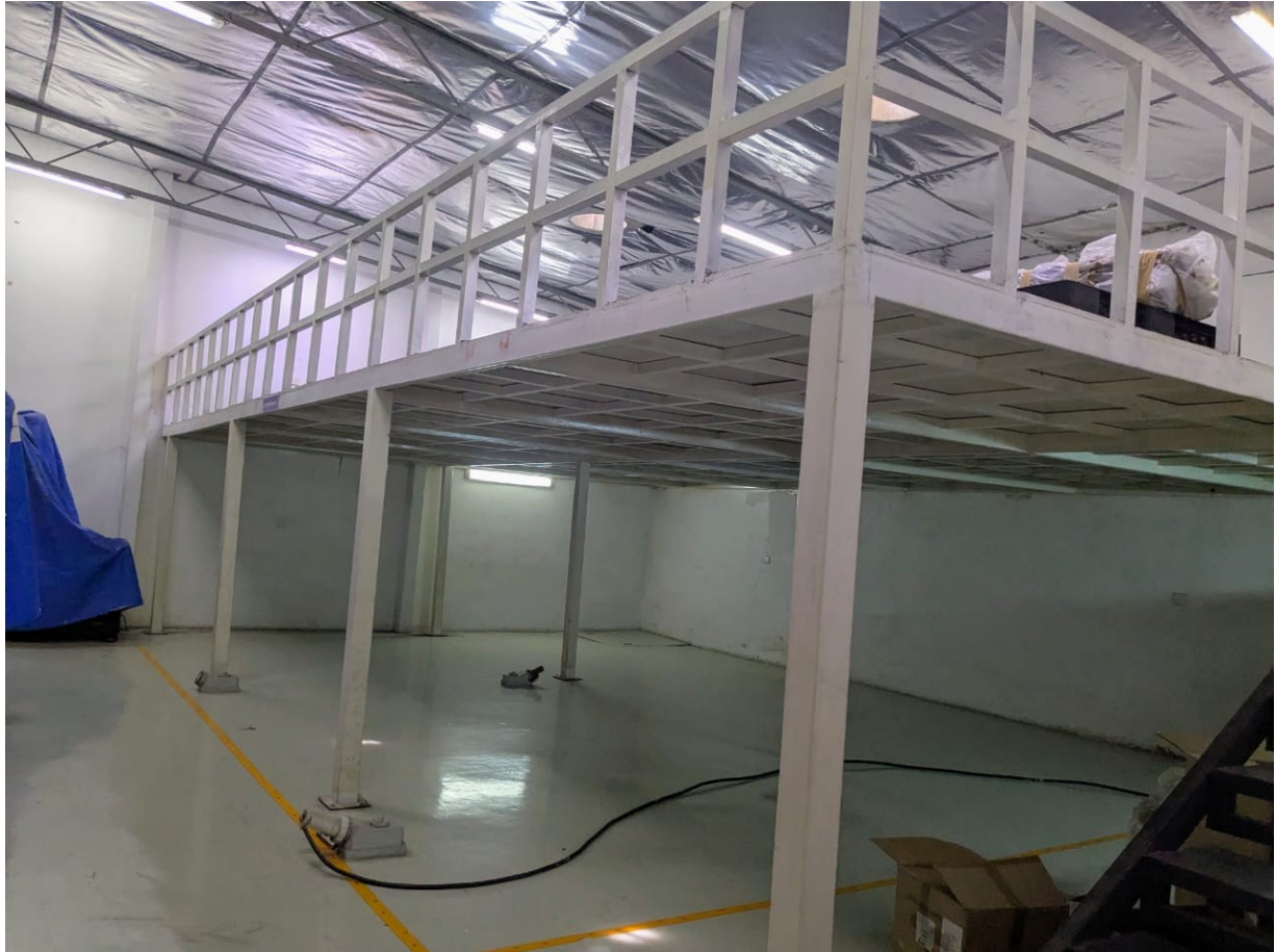
A picture which shows a shelf for storage of medicines
